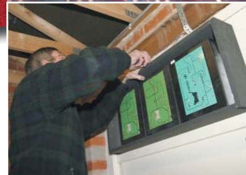
Upgrading an existing system.
